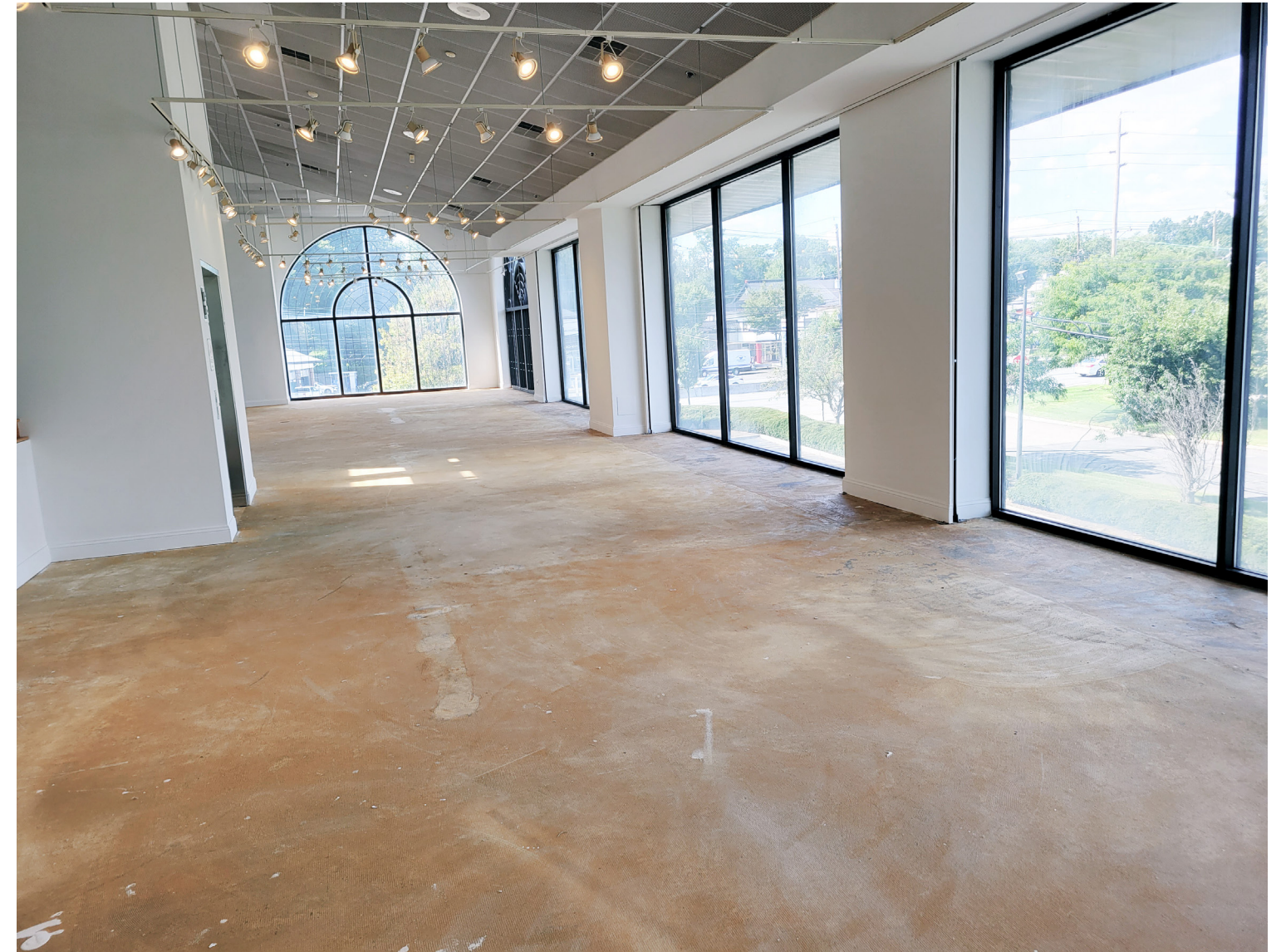
INTERIOR SECOND FLOOR
