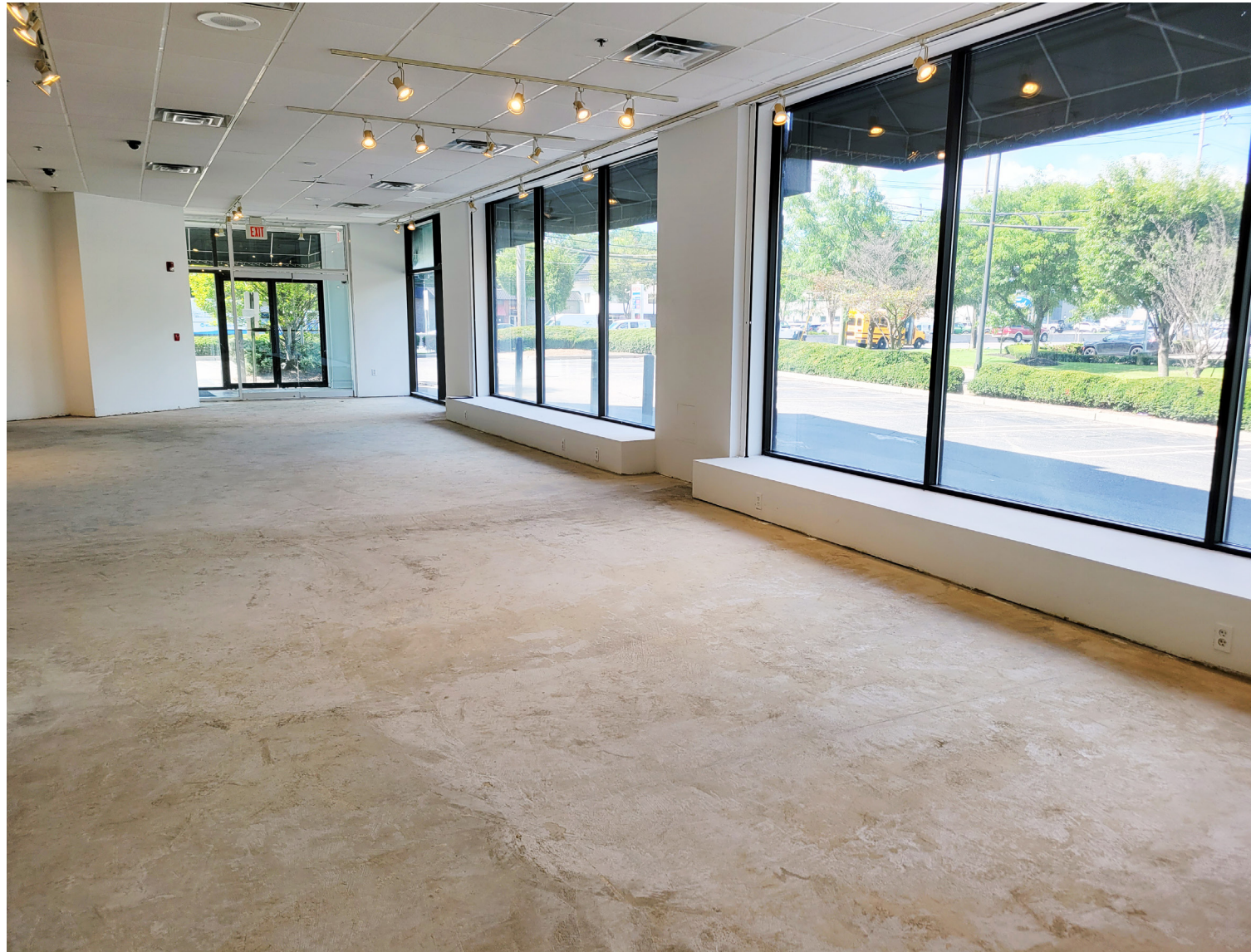
INTERIOR GROUND FLOOR
