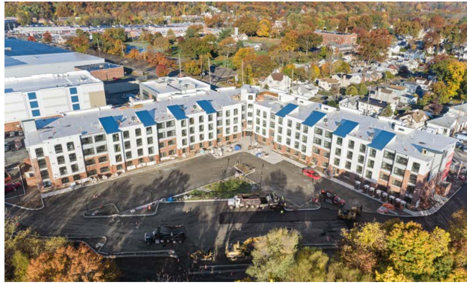
UNDER CONSTRUCTION - DELIVERY Q1 2023
