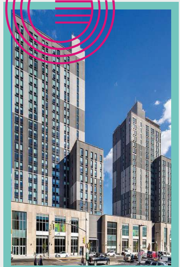
ARCHER GREEN APARTMENTS
