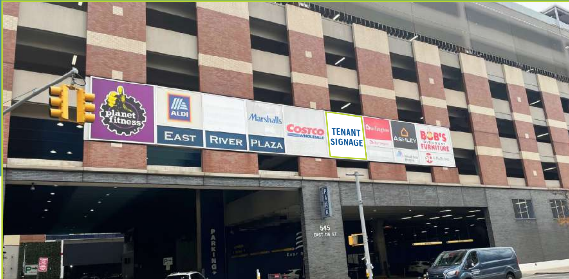
Signage at garage entrance
