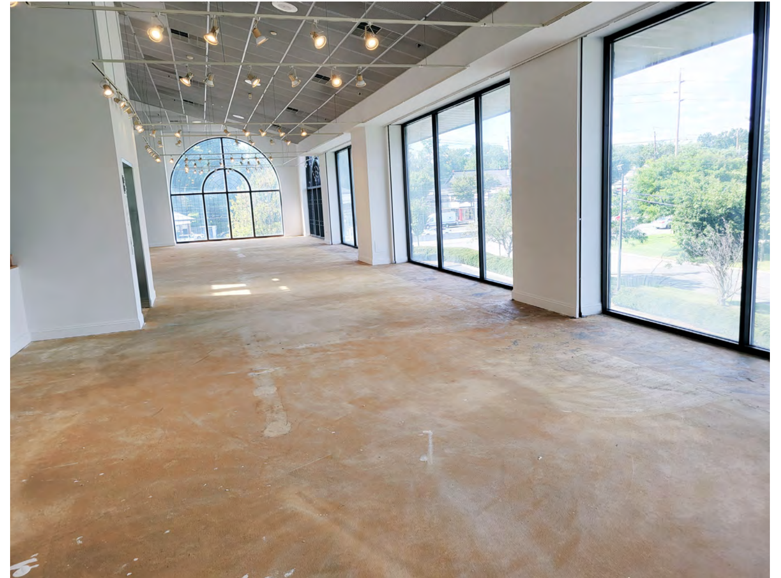
INTERIOR SECOND FLOOR
