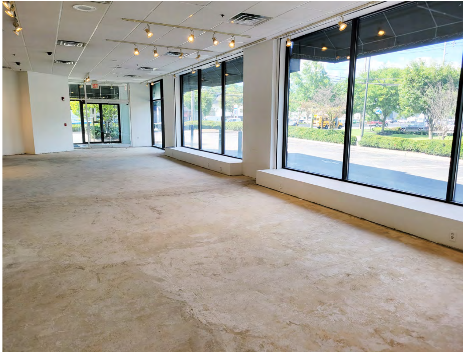
INTERIOR GROUND FLOOR
