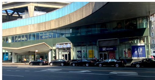
BROADWAY LOOKING ACROSS FROM THE SPACE
