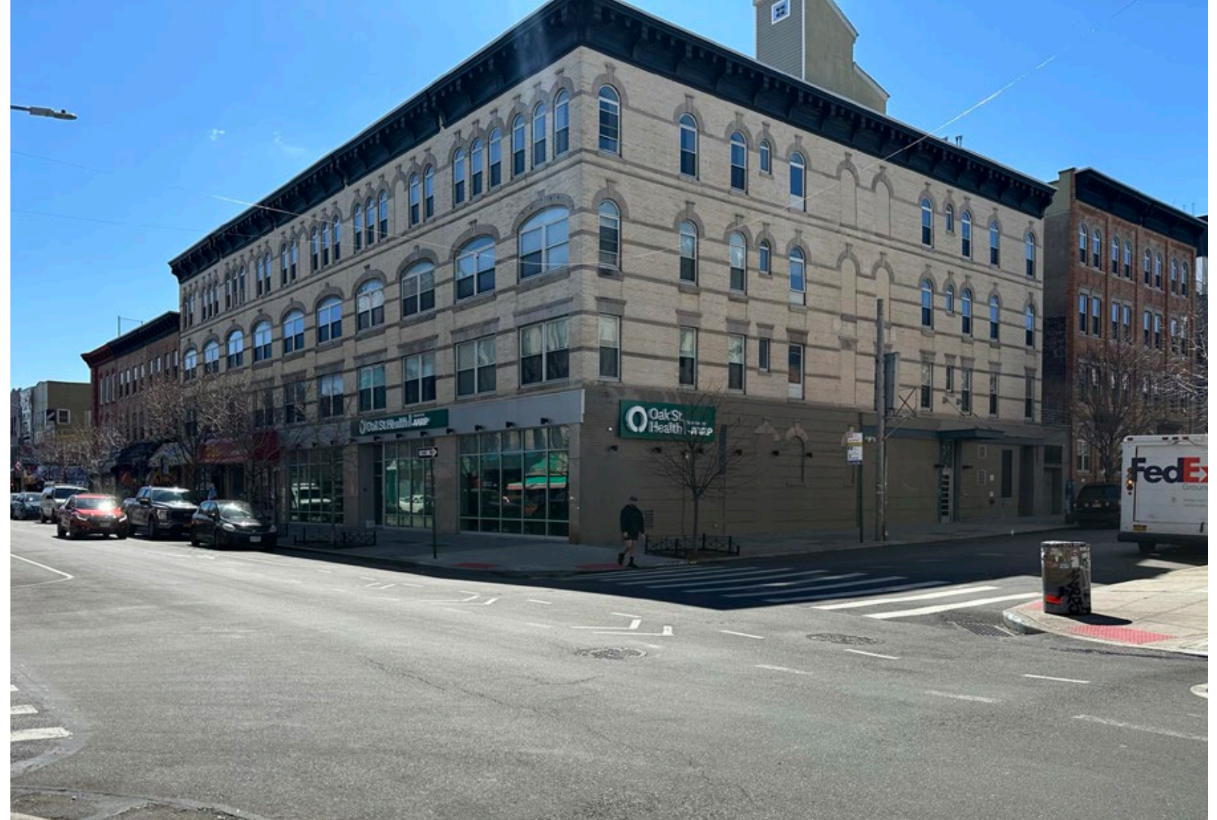
NEWLY OPENED OAK STREET HEALTH ACROSS THE STREET FROM SITE
