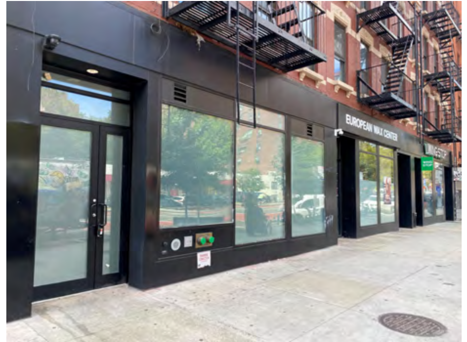
View looking west, with co-tenants at the building
